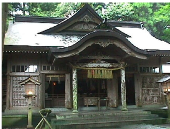
a. Principal shrine building.
