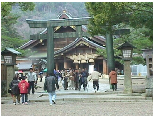
6. Frontal view of the oracle building.
